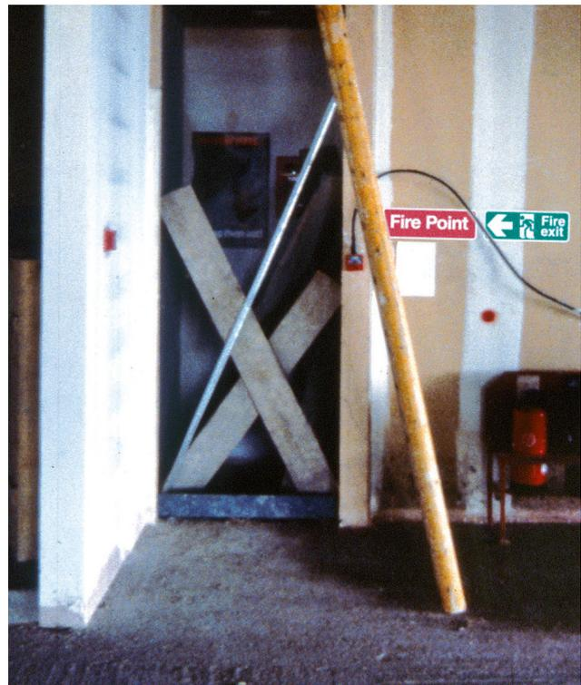
**Figure 9** Avoid creating dead ends and misleading fire exit signage
