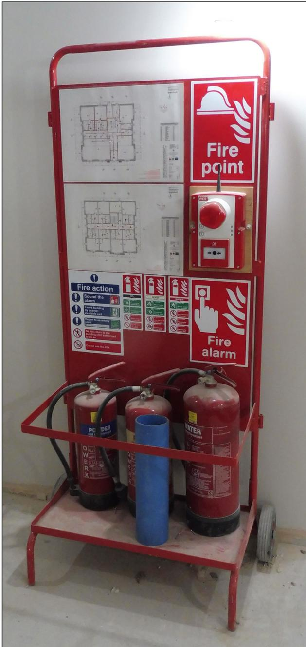
**Figure 16** An example of an interconnected alarm and fire extinguisher point in a refurbishment project. Most sites will require an interconnected alarm system (either wired or wireless)
