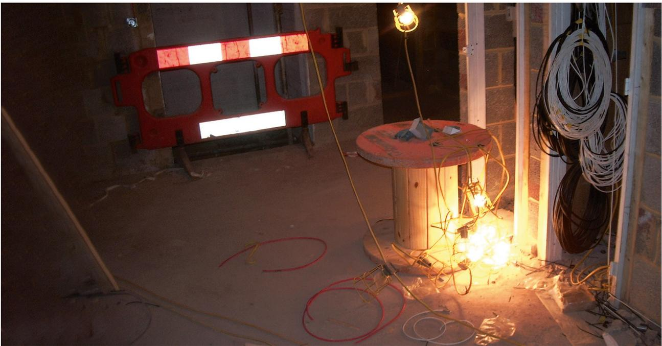
**Figure 4** Festoon lighting: poor positioning creates a potential fire risk
